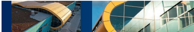
In the spirit of Feng Shui: Rhepanol hg on the shopping centre “Life” in Munich.
